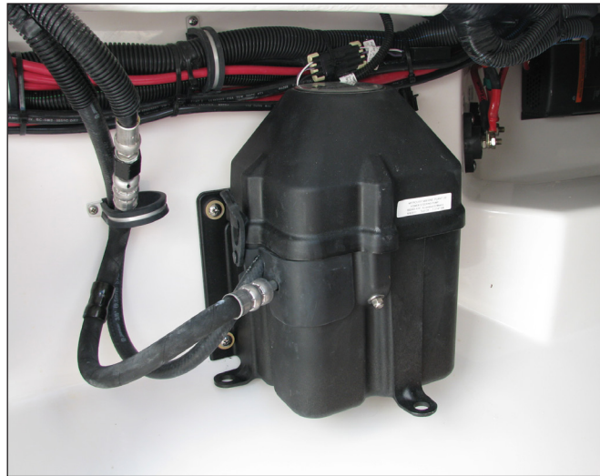
Power Steering Unit in Stern Bilge
