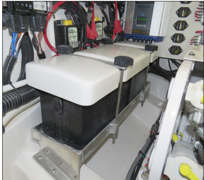
Port Engine Start Batteries in Aft Systems Compartment
