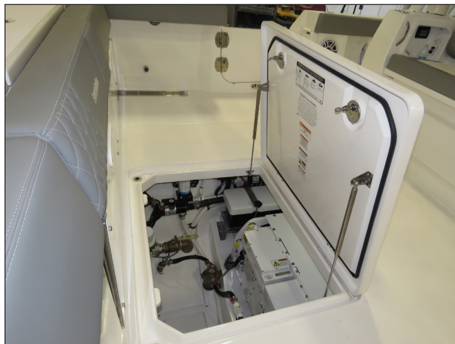
Aft Systems Compartment Hatch
