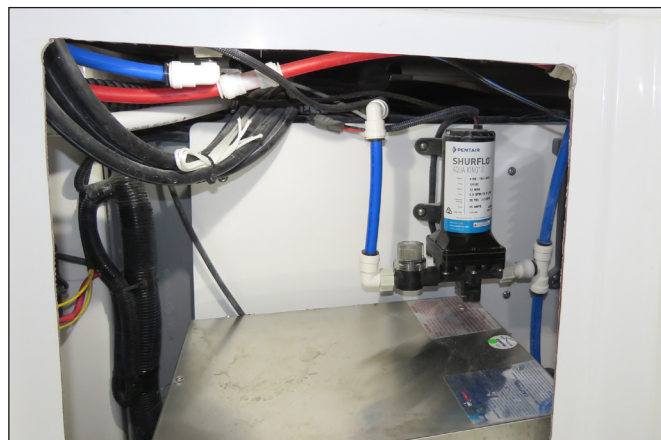
Lower Access Door & Forward Bilge Compartment
