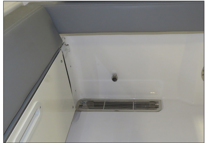
Typical Scupper Drains & Drain Rail
