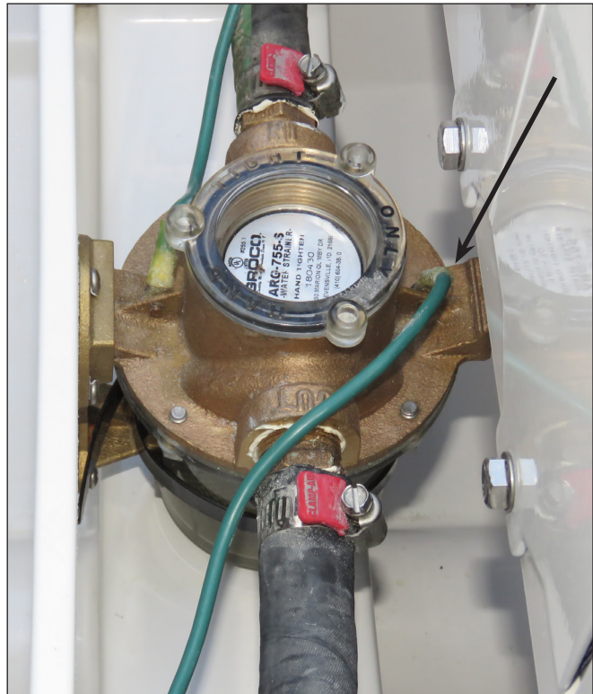
Typical Sea Strainer Bonding Wire
