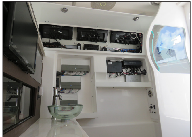
Upper Helm Access Compartment
