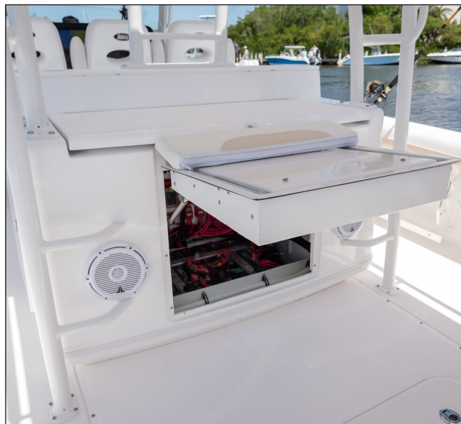
Electrical Systems Compartment Hatch
