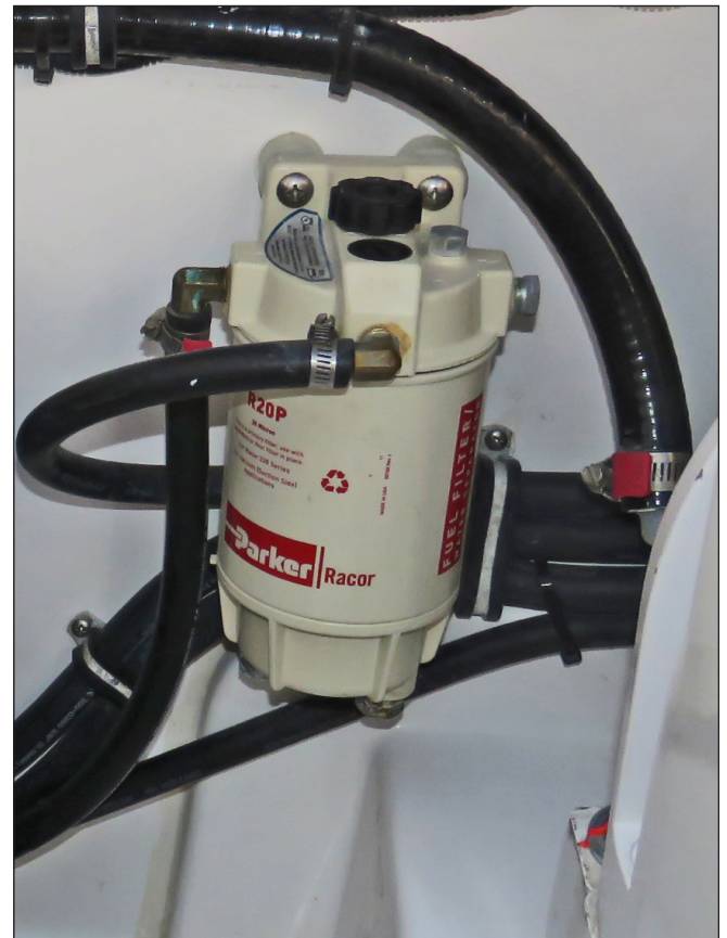
Generator Water Separator Fuel Filter
