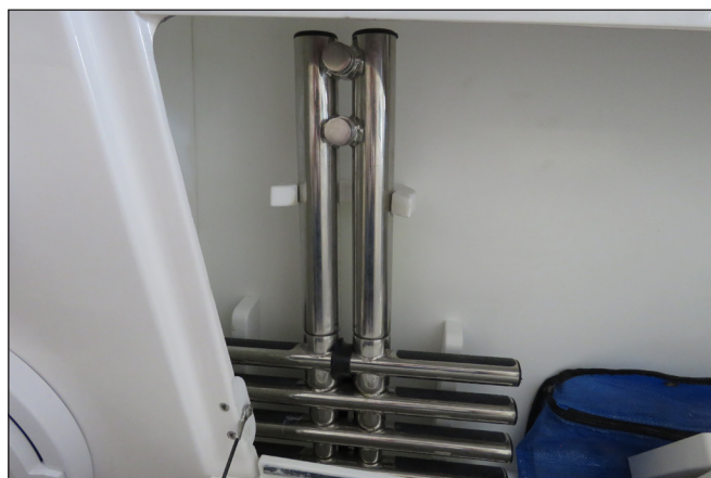
Boarding Ladder in Storage Compartment
