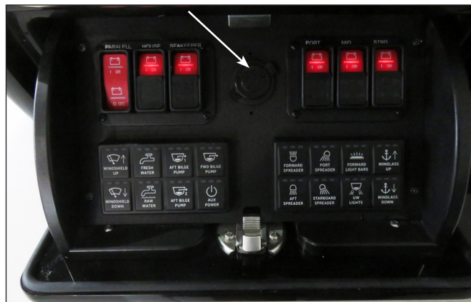
12 Volt Receptacle in Helm Switch Panel
