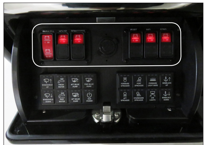
Helm Battery Switch Panel
