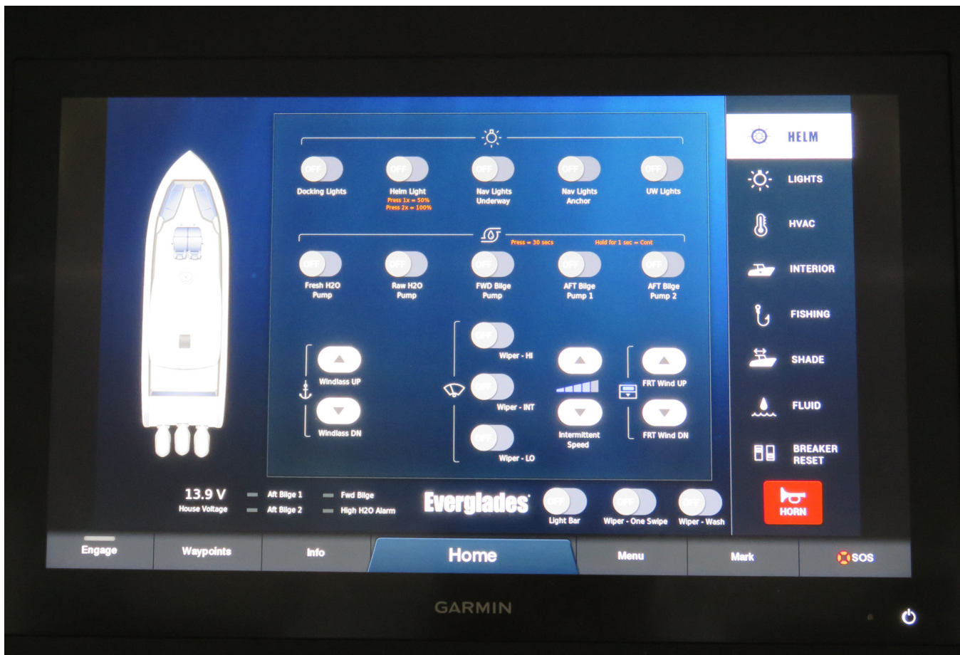
Typical Switches in the Helm Switch Touch Screen Display
