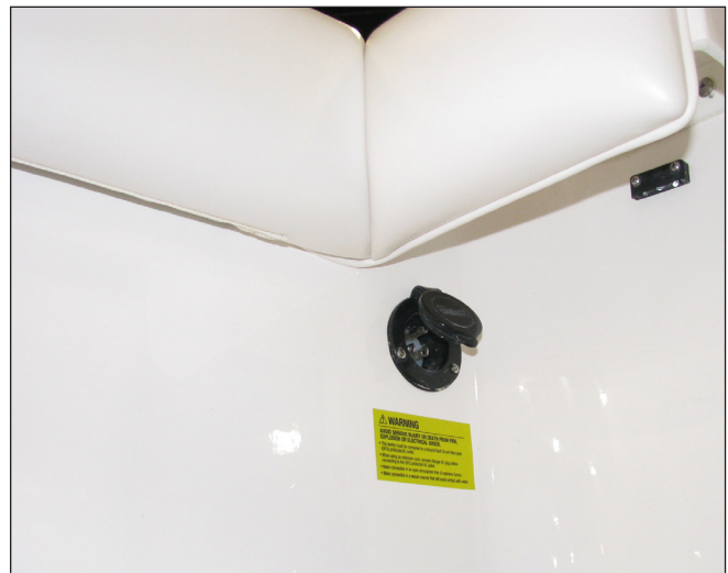
Shore Power Inlet Connection
