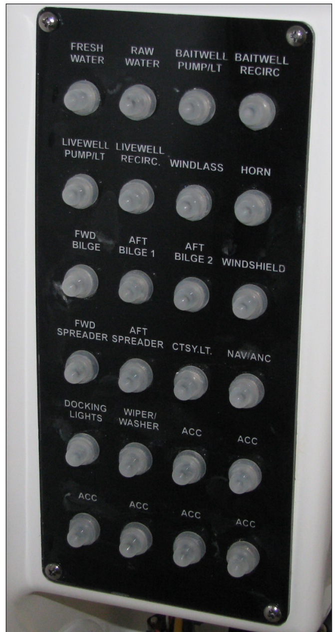
Head Compartment Circuit Breaker Panel
