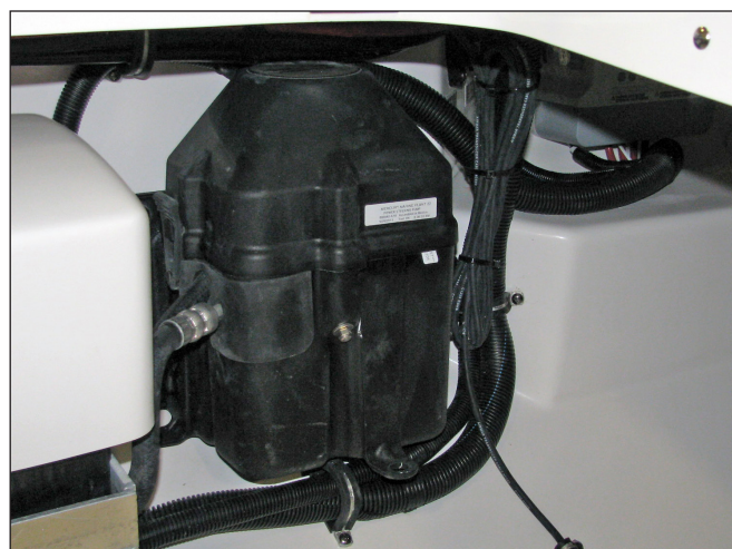
Power Steering Unit in the Systems Compartment
