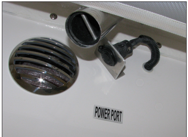
Typical Power Port
