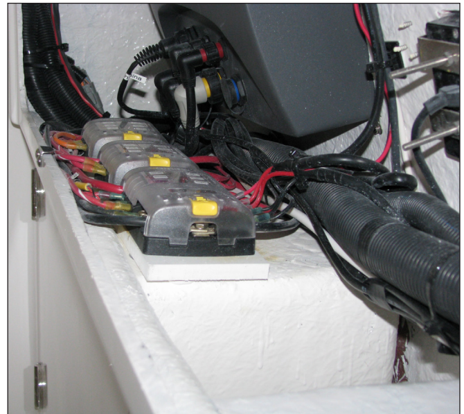
Electronics and Accessory Fuse Panels Behind Helm
