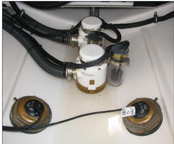
Typical Aft Bilge Pumps & Automatic Switches
