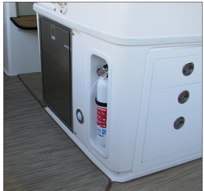
Port Prep Island Refrigerator & Fire Extinguisher
