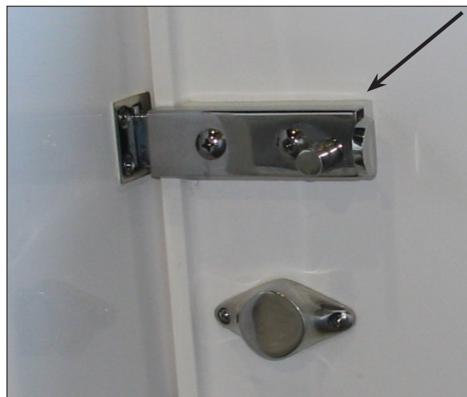
Utility Door Latch & Spring Loaded Safety Pin
