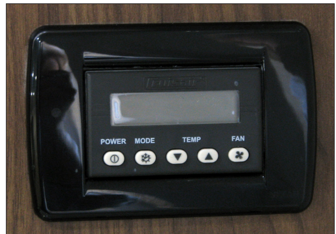
Cabin Air Conditioner Control Panel
