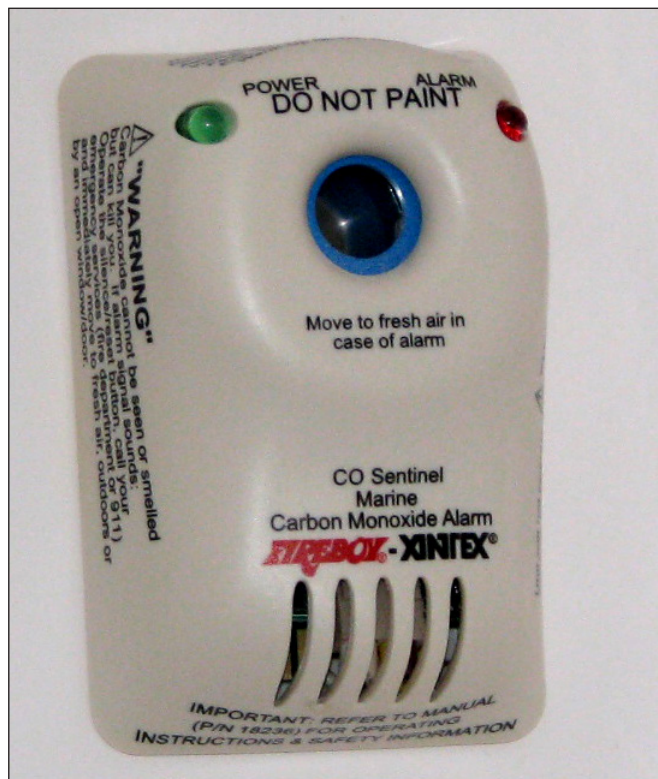
Typical Carbon Monoxide Detector & Alarm
