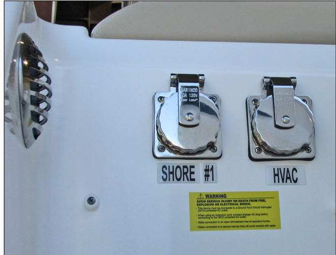
Shore Power Inlets 1 & 2/HVAC
