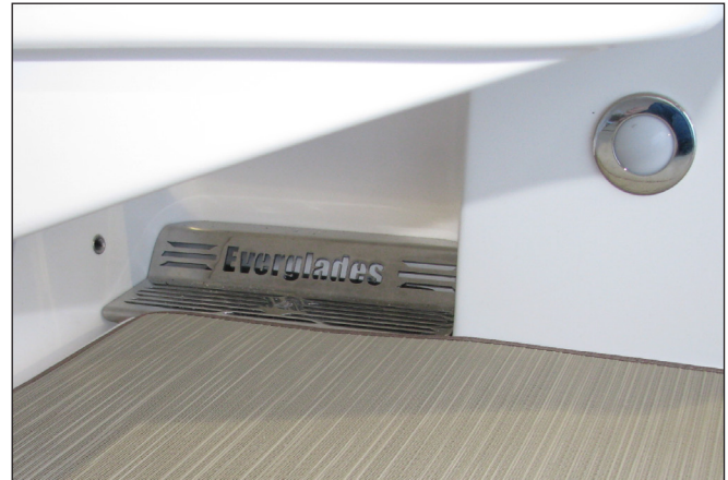
Typical Scupper Drains
