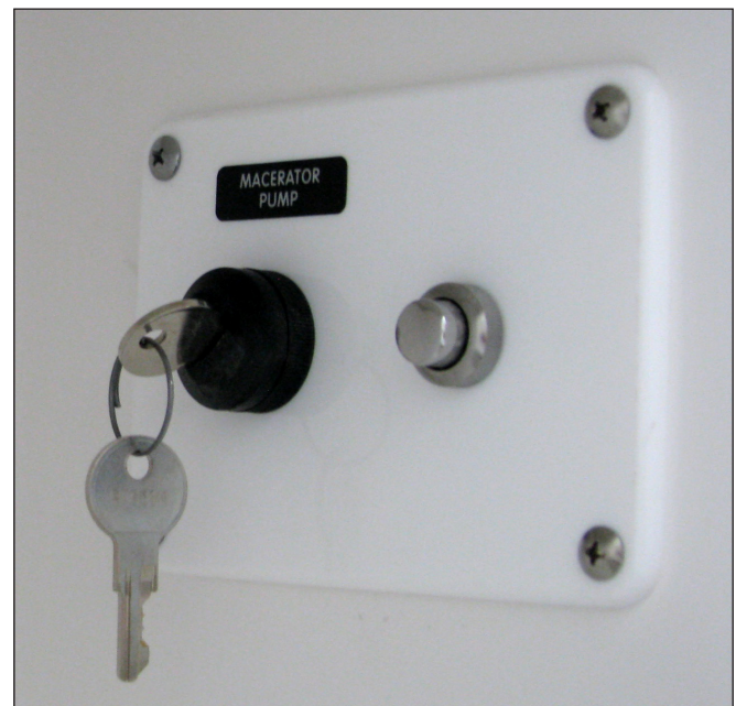
Waste Discharge Switch Panel
