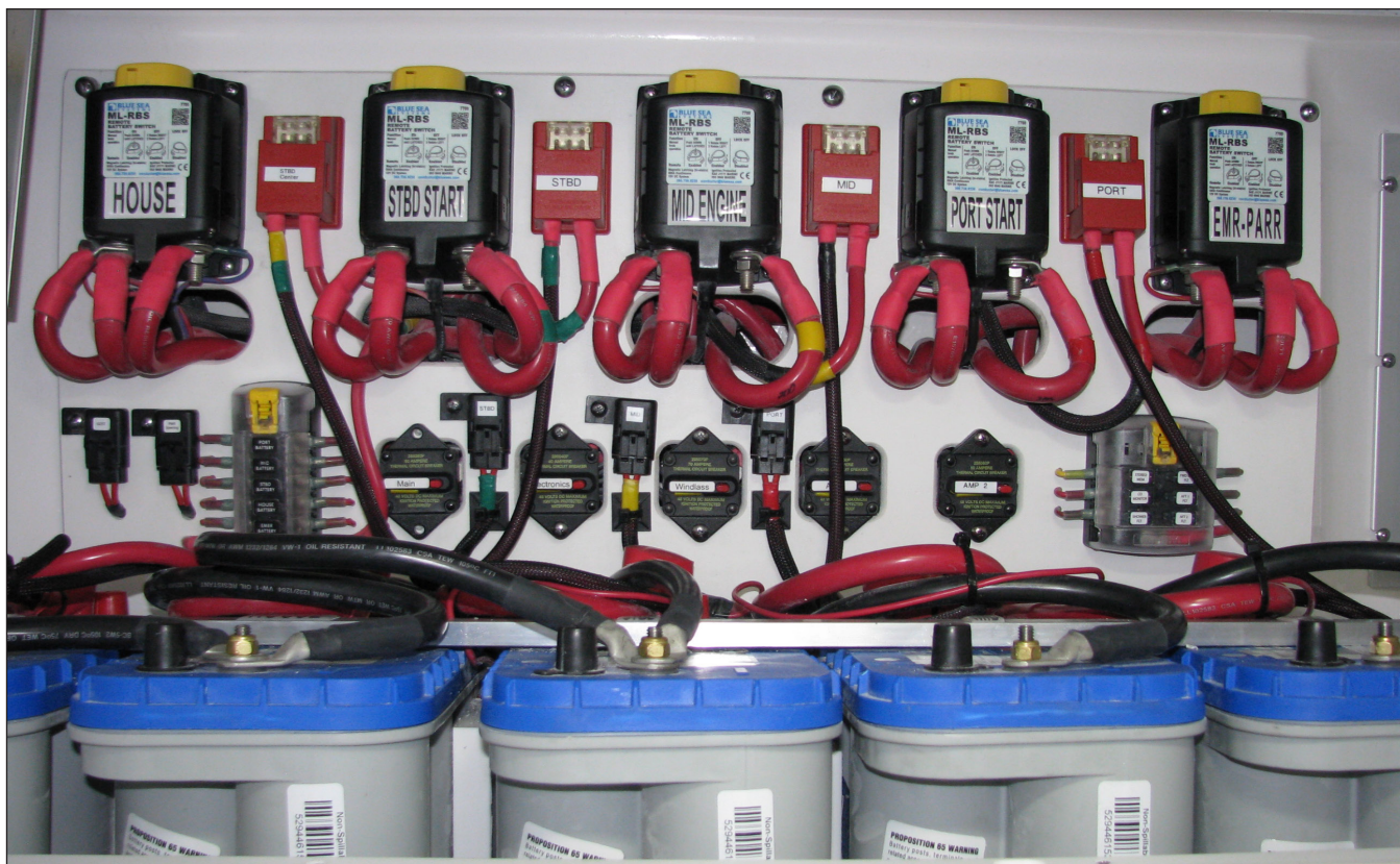
Battery Switches, Main Circuit Breakers, Main Fuses, Fuse Panels & Continuous Power Fuse Panels
