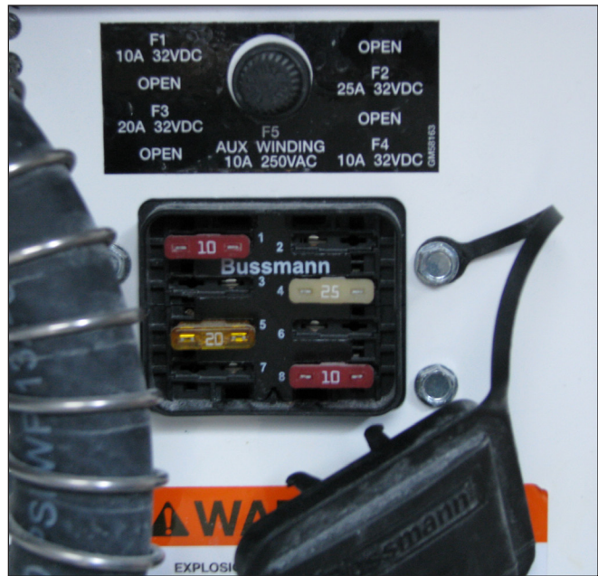
Typical Generator DC System Circuit Protection
