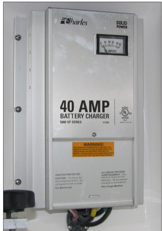
Typical Battery Charger
