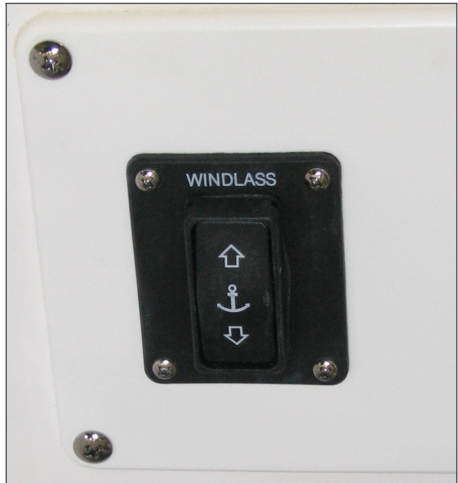
Windlass Switch in Rope Locker Near Windlass
