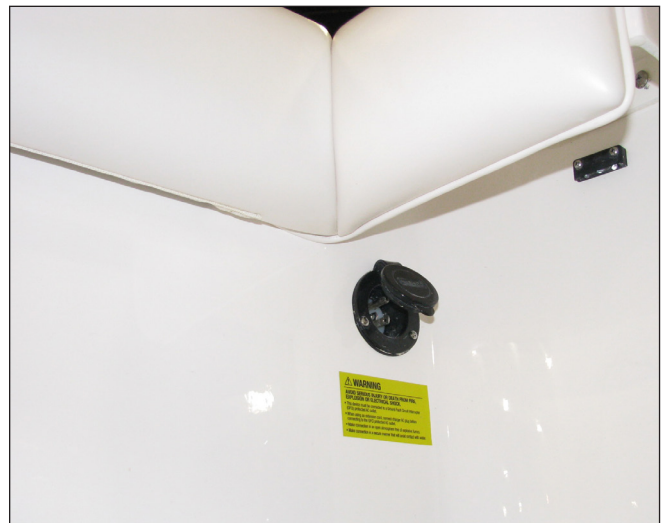
Shore Power Inlet Connection
