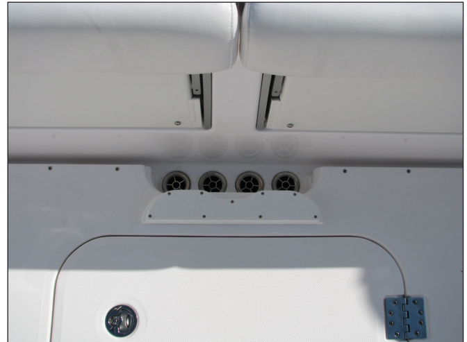
Typical Scupper Drains and Drain Rail
