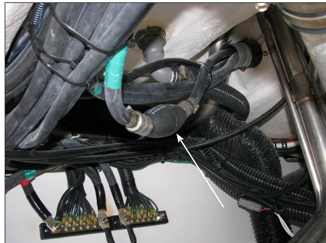
Primer Bulb at Rear Of Access Hatch
