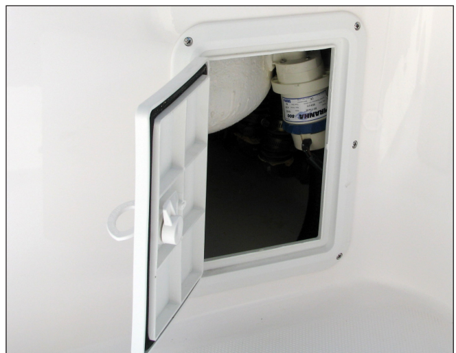
Livewell Recirculation Pump
