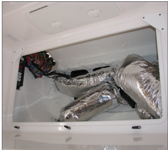
Helm Access Panel in Aft Cabin Headliner
