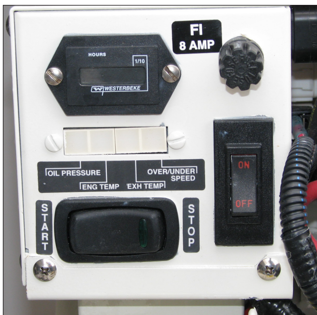
Generator Onboard Control Switch and Engine Monitor Fuses and Circuit Breaker
