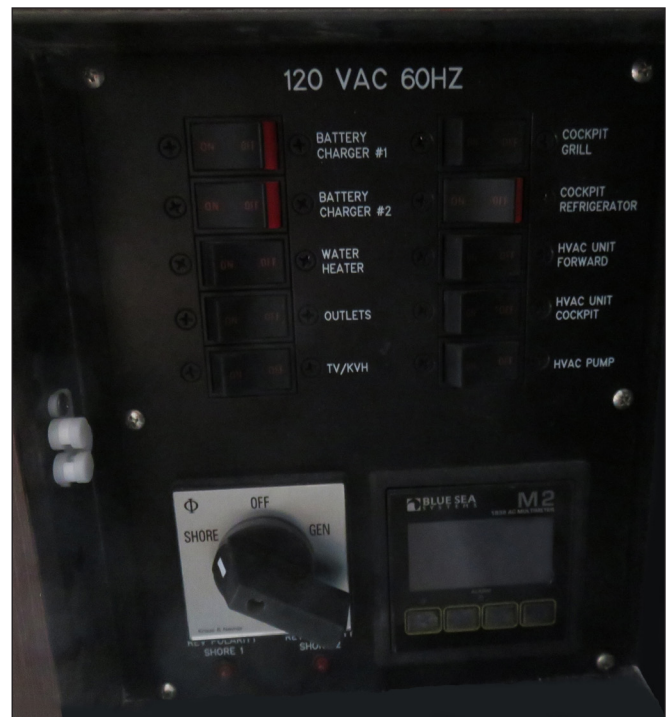
120 Volt AC Panel, SHORE/OFF/GENERATOR Selector Switch, Multimeter & Accessory Circuit Breakers
