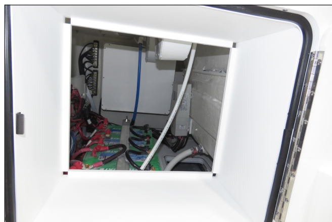
Access Panel Removed
