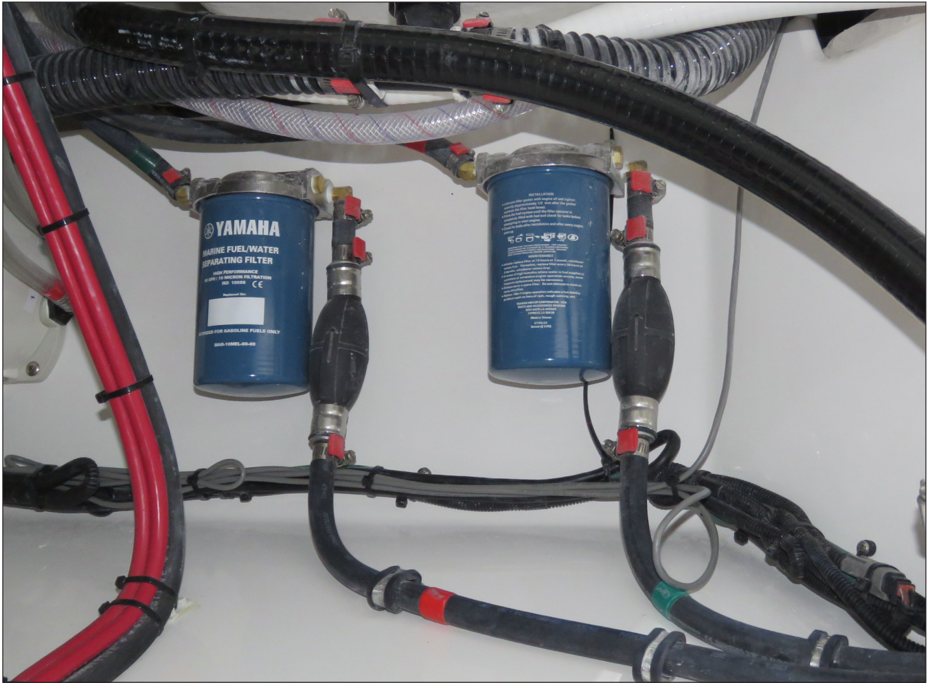
Typical Yamaha Engine Port & Starboard Engine Fuel Filters In Aft Systems Compartment
