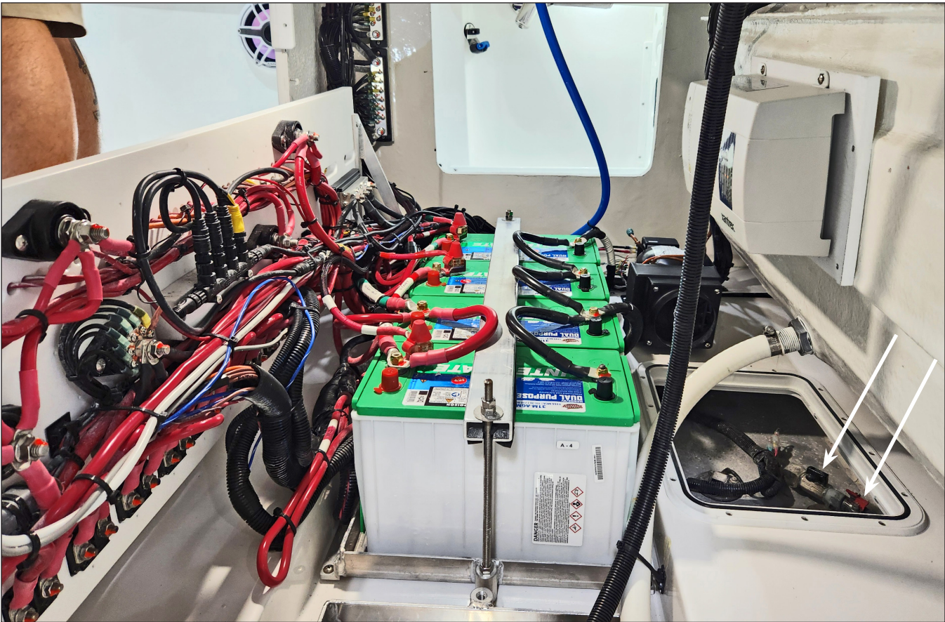
Fuel Valves & Fuel Gauge Sender Access Hatch In The Cockpit Sole In Battery Compartment
