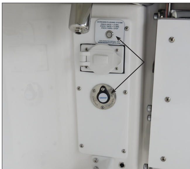
Typical Engine Flushing System Shore Hose Connection
