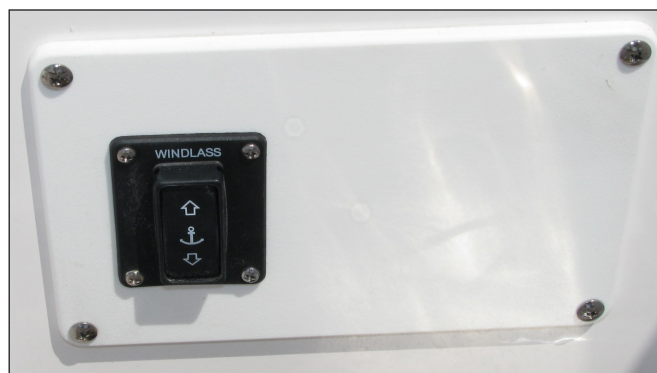
Windlass Switch in the Rear of the Rope Locker
