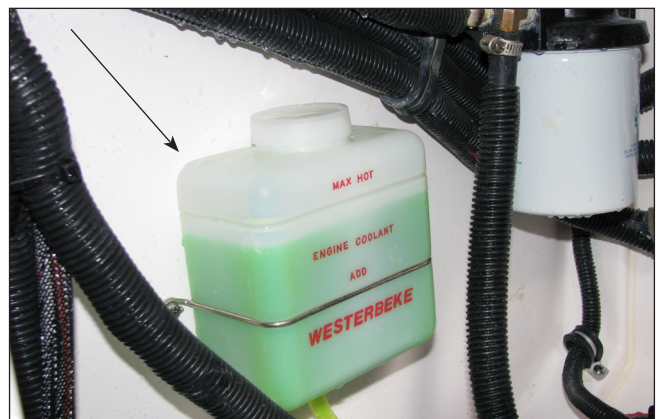
Generator Cooling System Expansion Tank
