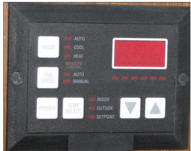
Air Conditioner Control Panel
