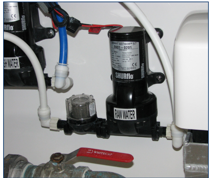
325 Pilot Raw Water Pump and Strainer
