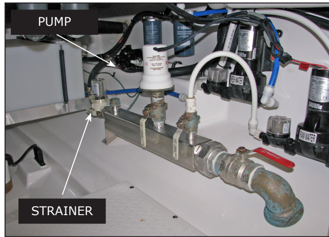
325 Pilot Air Conditioner Seawater Pump and Strainer
