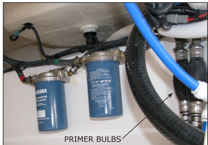
325 Pilot Fuel Filters and Primer Bulbs in Systems Compartment
