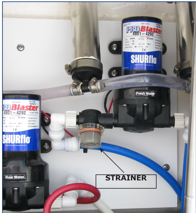
295 Pilot Fresh Water Pump & Strainer
