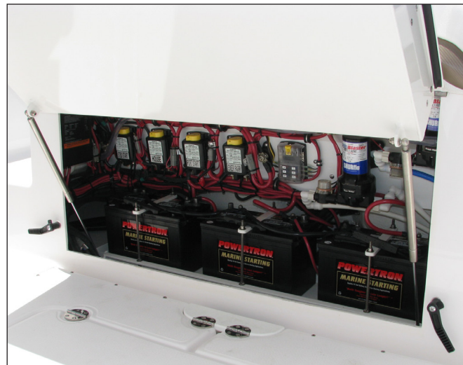
295 Pilot System Compartment and Batteries
