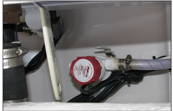
295 Pilot Baitwell Supply Pump and Seacock
