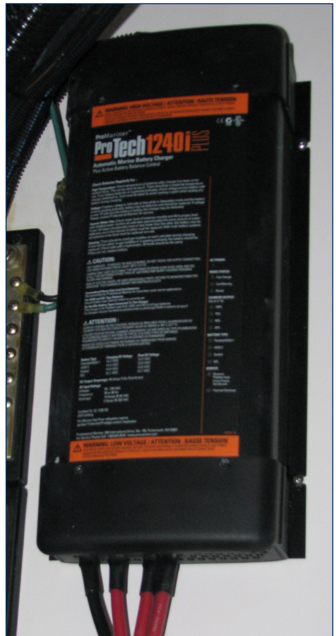
Typical Battery Charger
