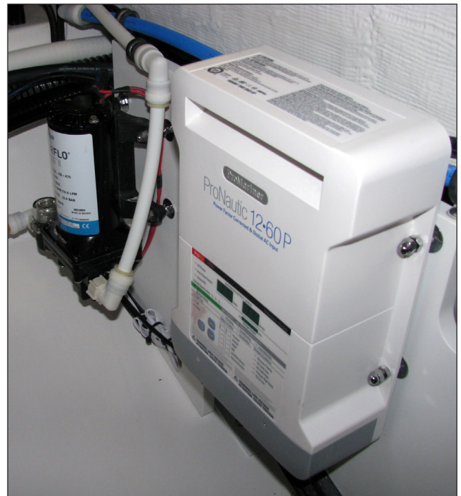
Typical Battery Charger
