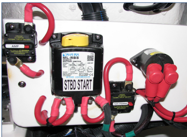
Typical Heavy Duty Circuit Breakers
