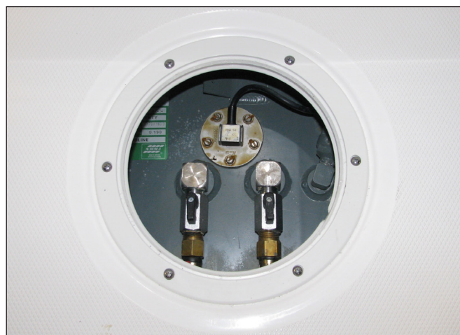
Typical Round Access Hatch In Cockpit
