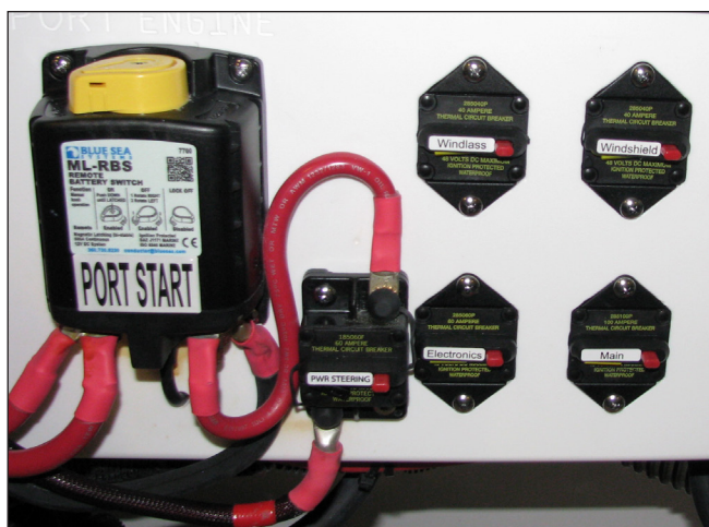
Typical Heavy Duty Circuit Breakers
