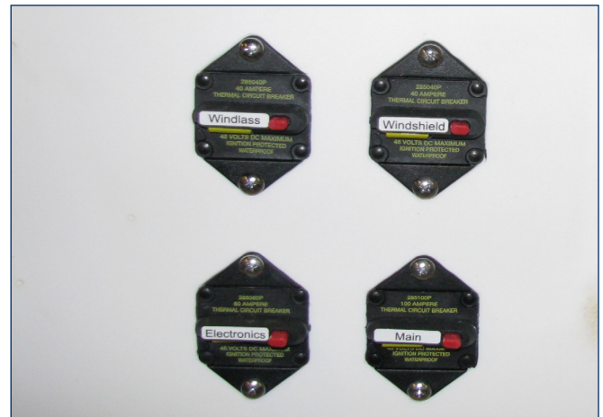
Typical Heavy Duty Circuit Breakers
