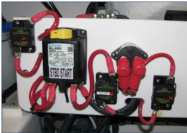
Typical Heavy Duty Circuit Breakers
