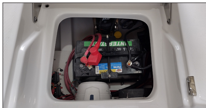
Starboard Battery Location
