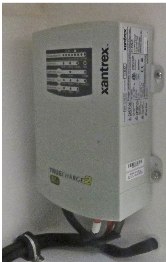
Typical Battery Charger
