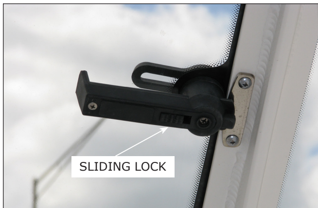
Twist Action Cam Lever and Sliding Lock
