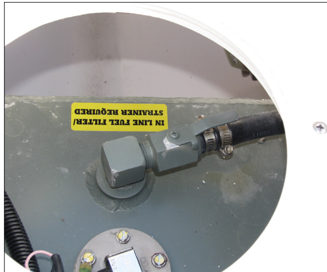
Typical Fuel Shutoff Valve
