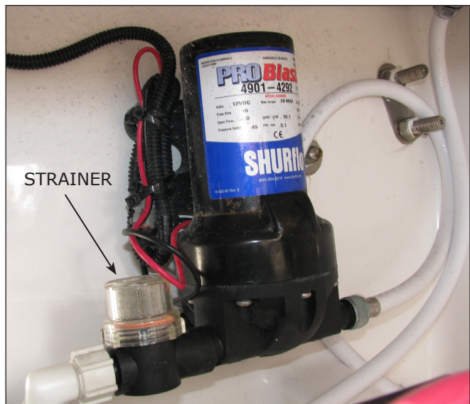
Typical Fresh Water Pump and Strainer
