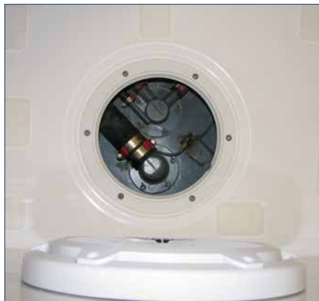
Fuel Fill & Vent Hose Connections
