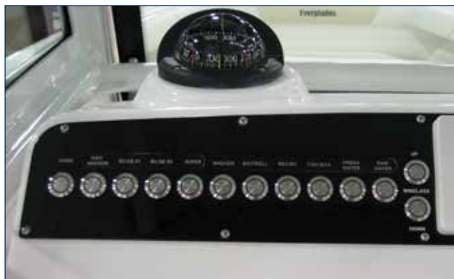
Port Side Helm Switches
