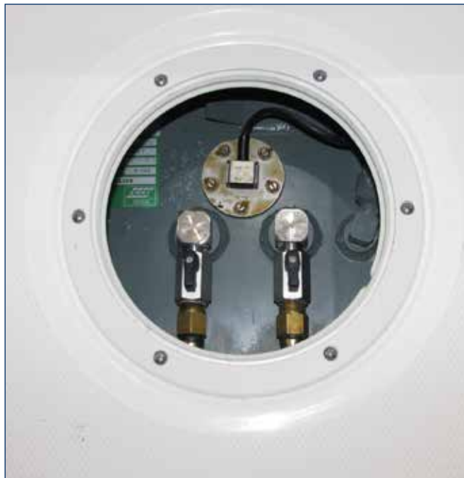
Fuel Withdrawal Valves & Tank Sending Unit
