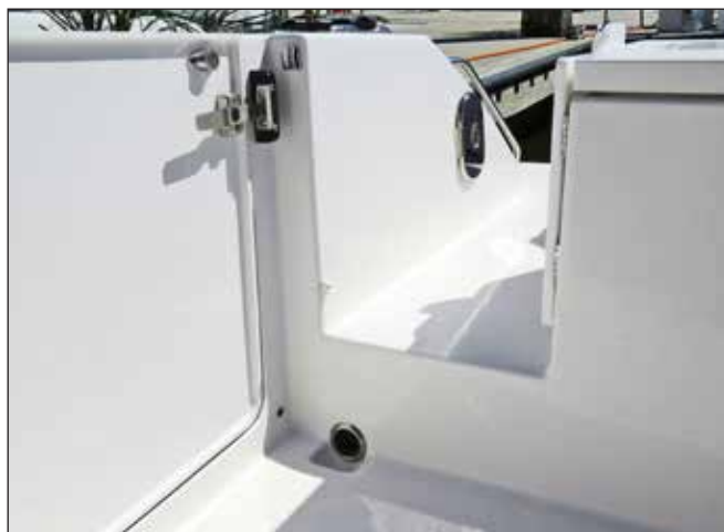
Typical Scupper Drains
