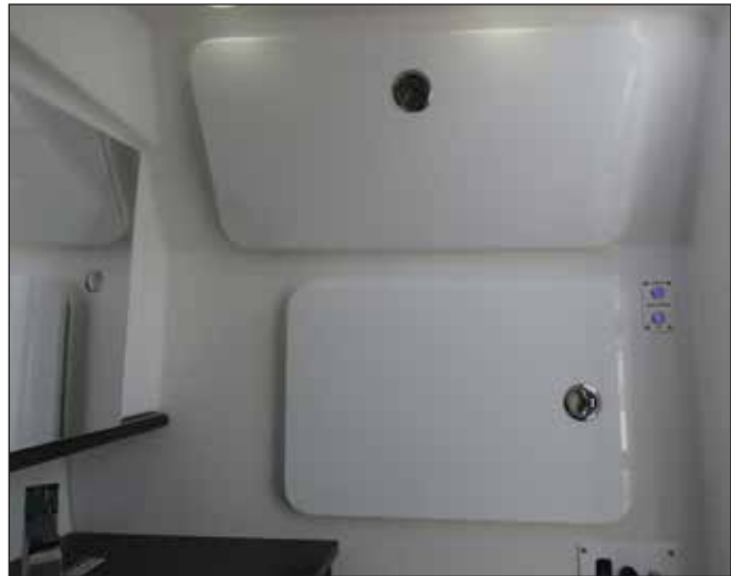
Access Hatches in Rear Bulkhead
