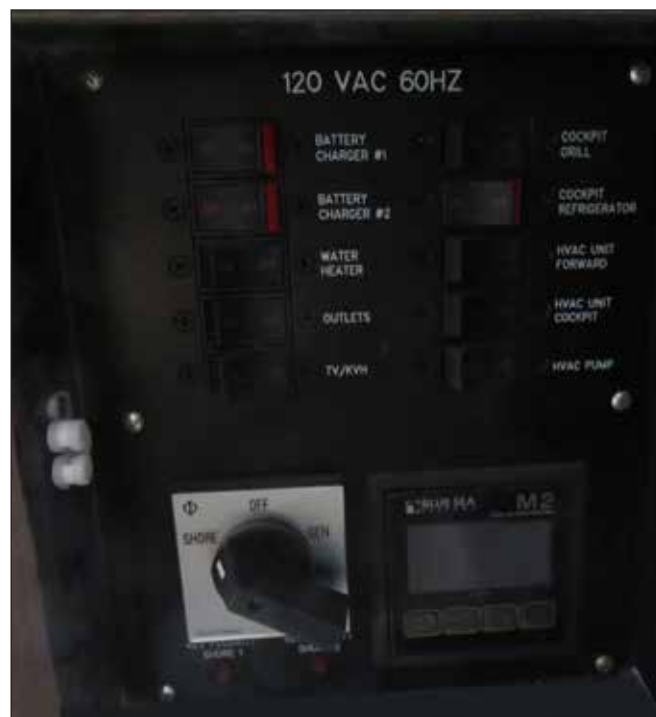
120 Volt AC Panel, SHORE/OFF/GENERATOR Selector Switch, Multimeter & Accessory Circuit Breakers
