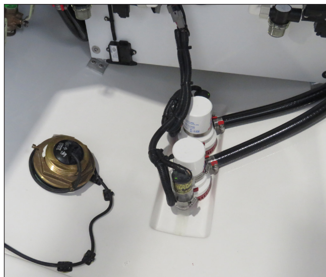
Aft Bilge Pumps & Automatic Switches
