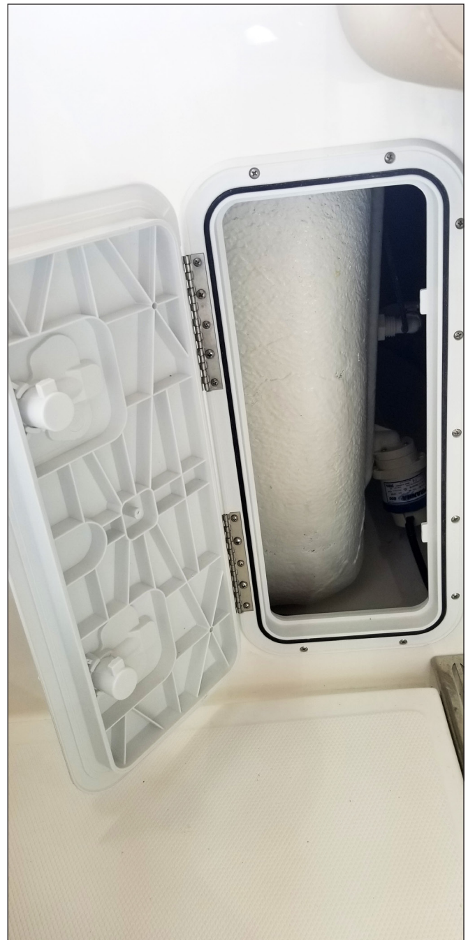
Baitwell Recirculating Pump Access Door
