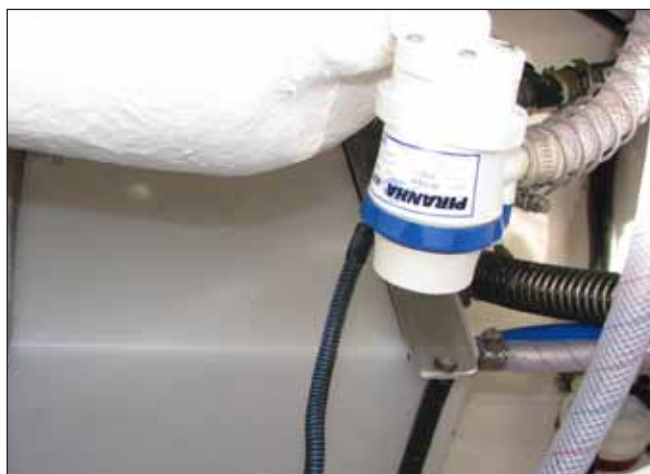
Baitwell Recirculation Pump
