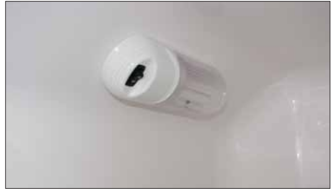
12 Volt Light in Head Compartment
