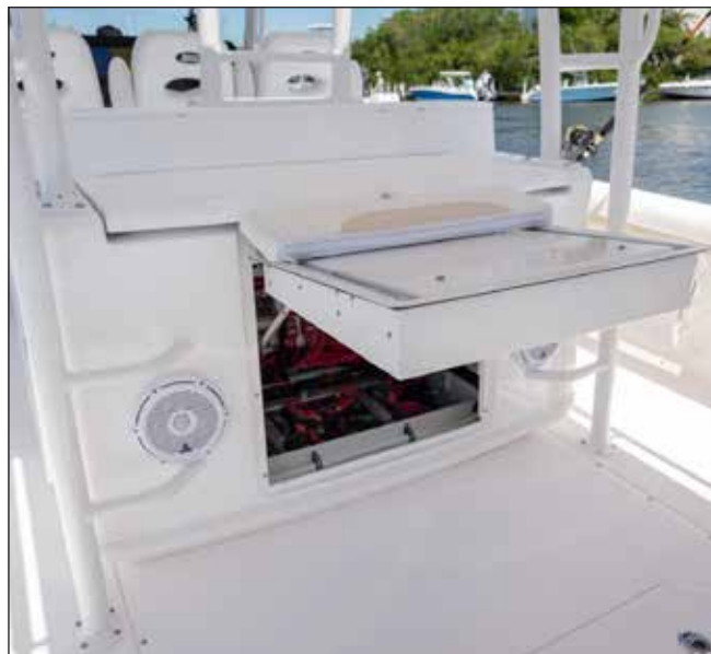
Electrical Systems Compartment Hatch
