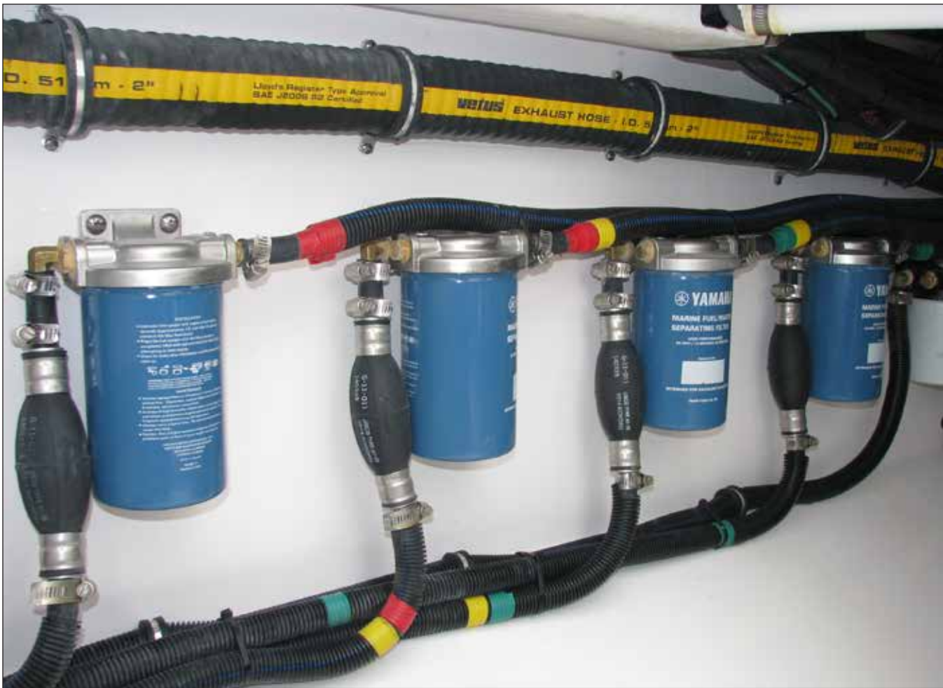
Typical Yamaha Quad Engine Fuel Filters & Primer Bulbs
