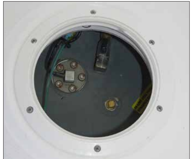
Fuel Gauge Sender & Withdrawal Valve
