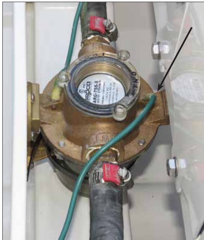
Typical Sea Strainer Bonding Wire
