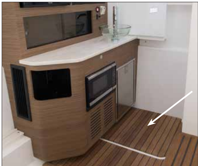
Removable Cabin Floor Panel Remove To Access Forward Bilge Pump & Drain Sump Pump
