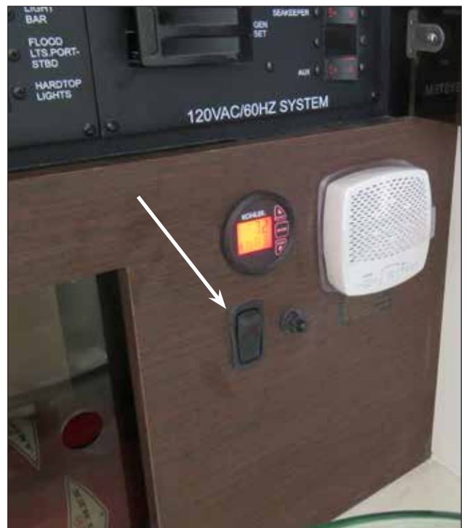
Cabin Bilge Blower Switch
